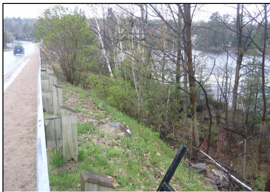
Plate 11: View south on 169 and downslope into site of Bala No. 2 foundation . Level ground at bottom has potential for industrial remains.
