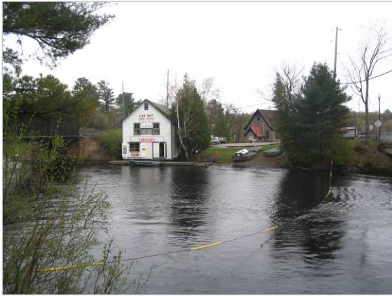
Plate 9: Land between boathouse and 169 has potential. Excavation passes across between trees and under highway.
