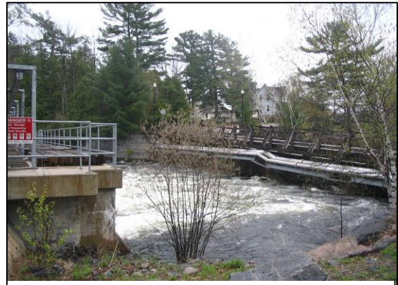
Plate 2: Dam and Bala Falls Rd. bridge over South Bala Falls.
