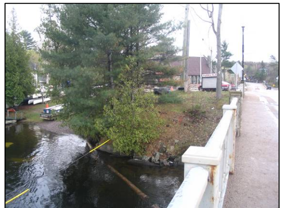
Plate 4: Highway 169 bridge over North Bala Falls channel showing an area of potential near trees on left.
