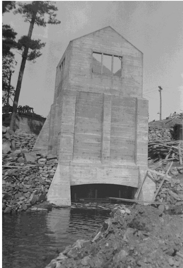
Photograph 12: Bala #2 Generating Station under construction showing tail race and rip-rap rock placed on both sides of the building, 1924.
