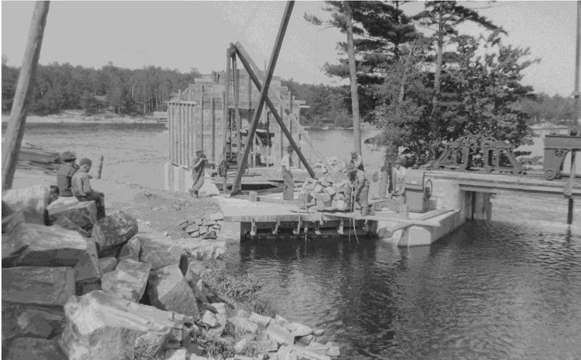
Photograph 11: Bala #2 Generating under construction showing head race and North Channel Dam on right, 1924.
