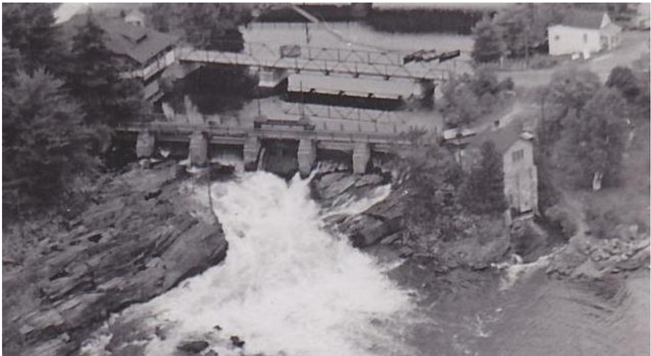
Image 10: Bala #2 Generating Station pre 1956
