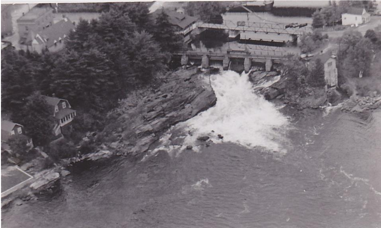
Image 5: Bala #2 Generating Station pre 1956
