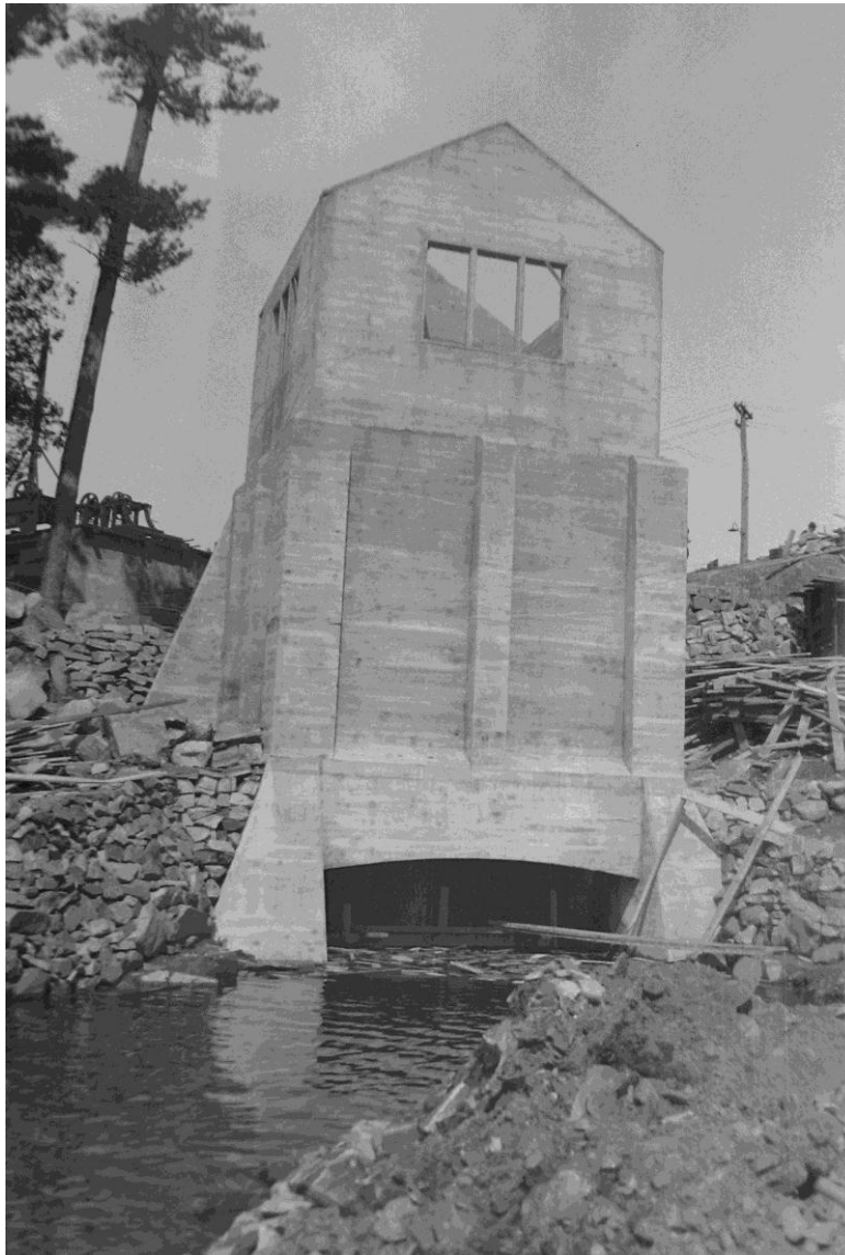
Image 6: Bala #2 Generating Station under construction showing tail race, 1924.
