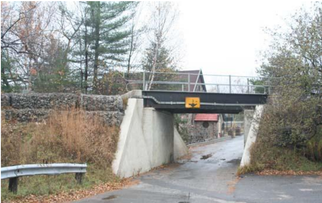
Image 16: The single lane Ball Road underpass with low headroom under the Canadian Pacific with the Presbyterian church in rear, 2009.
