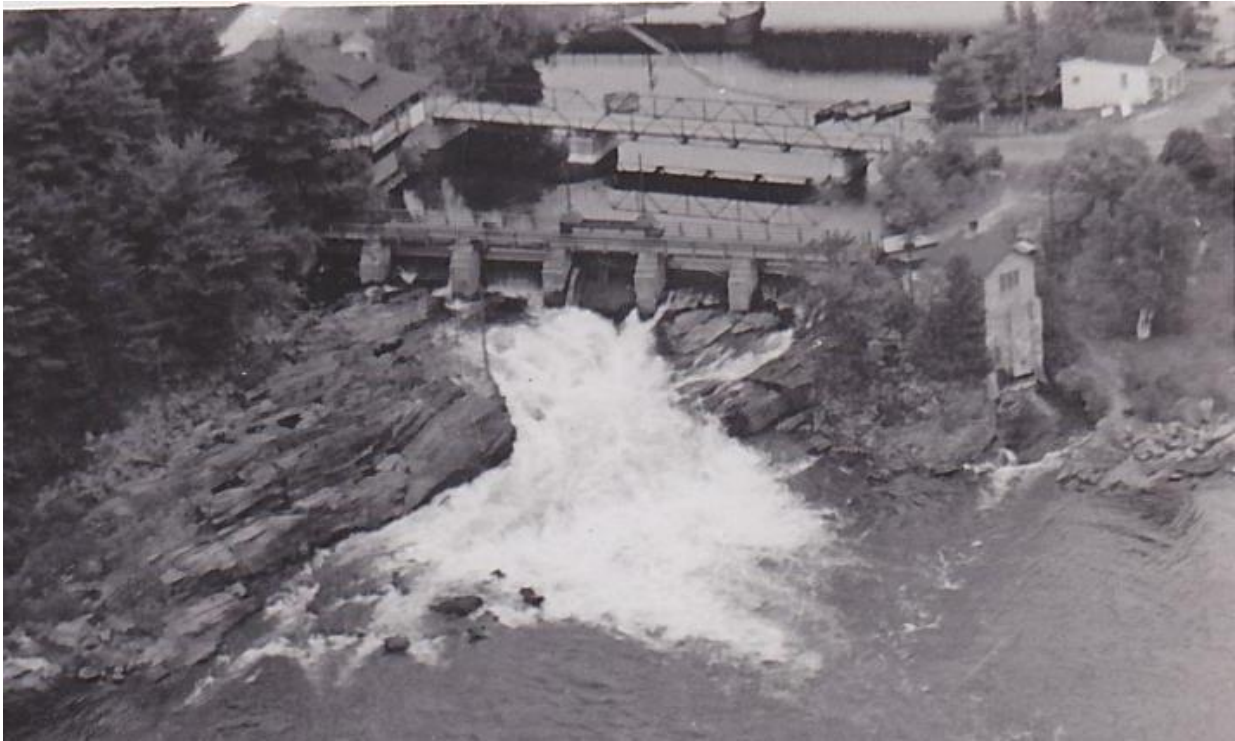
Photograph 2: Bala #2 Generating Station at the North Bala Falls, pre 1956.
