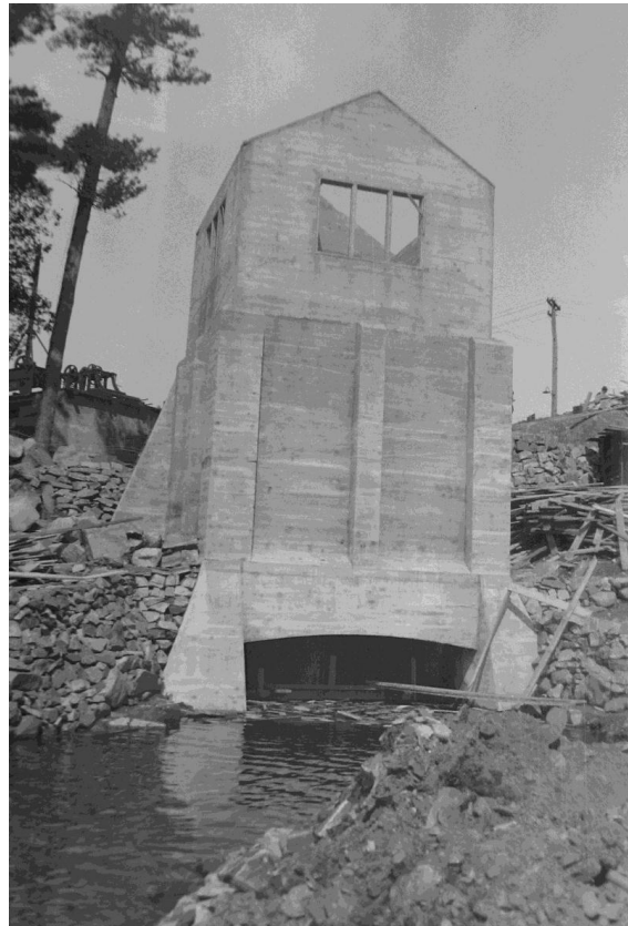
Photograph 12: Bala #2 Generating Station under construction showing tail race and rip-rap rock placed on both sites of the building, 1924.
