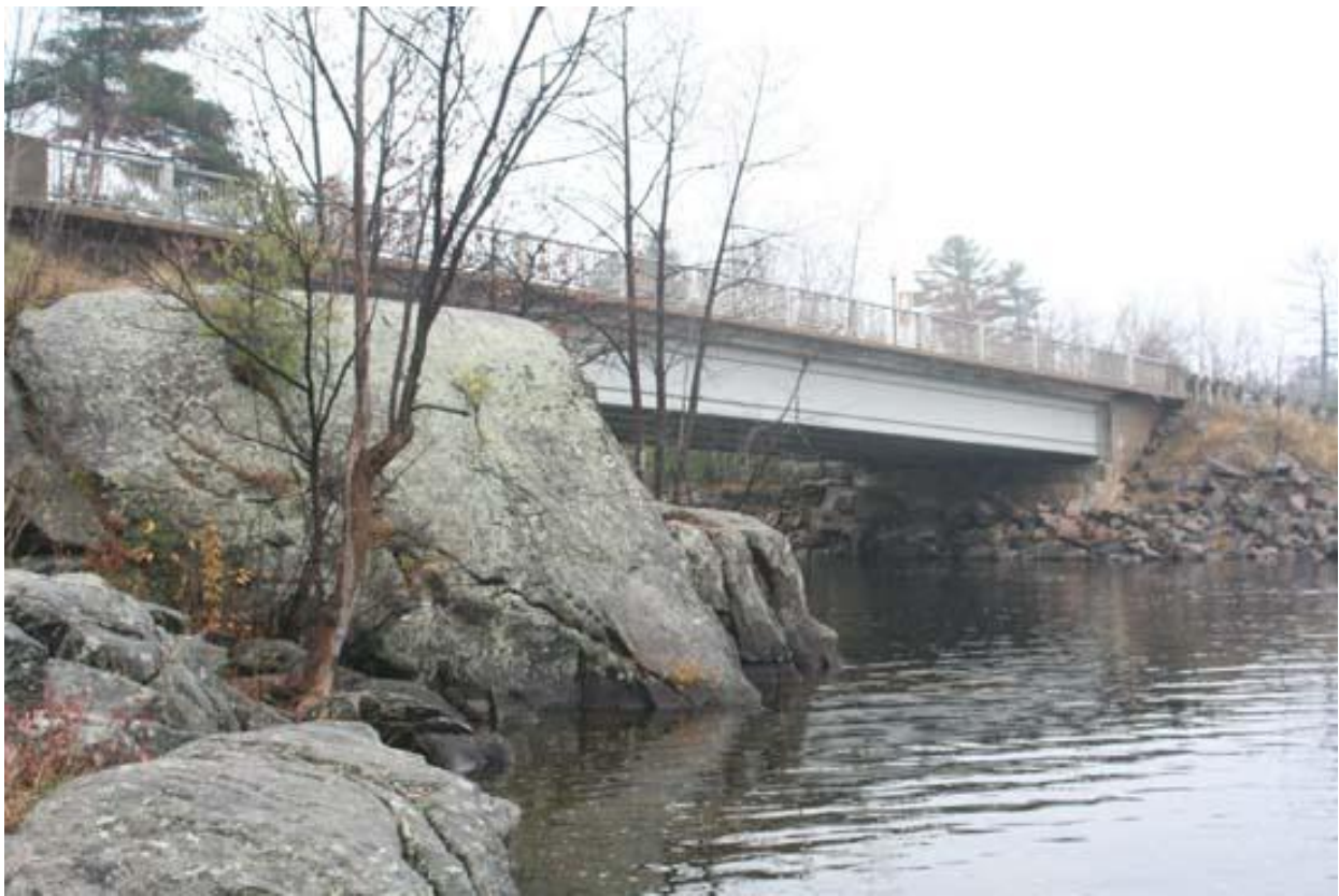
Image 12: South Channel bridge showing bedrock of original shoreline on left and filled shore on right, 2009.
