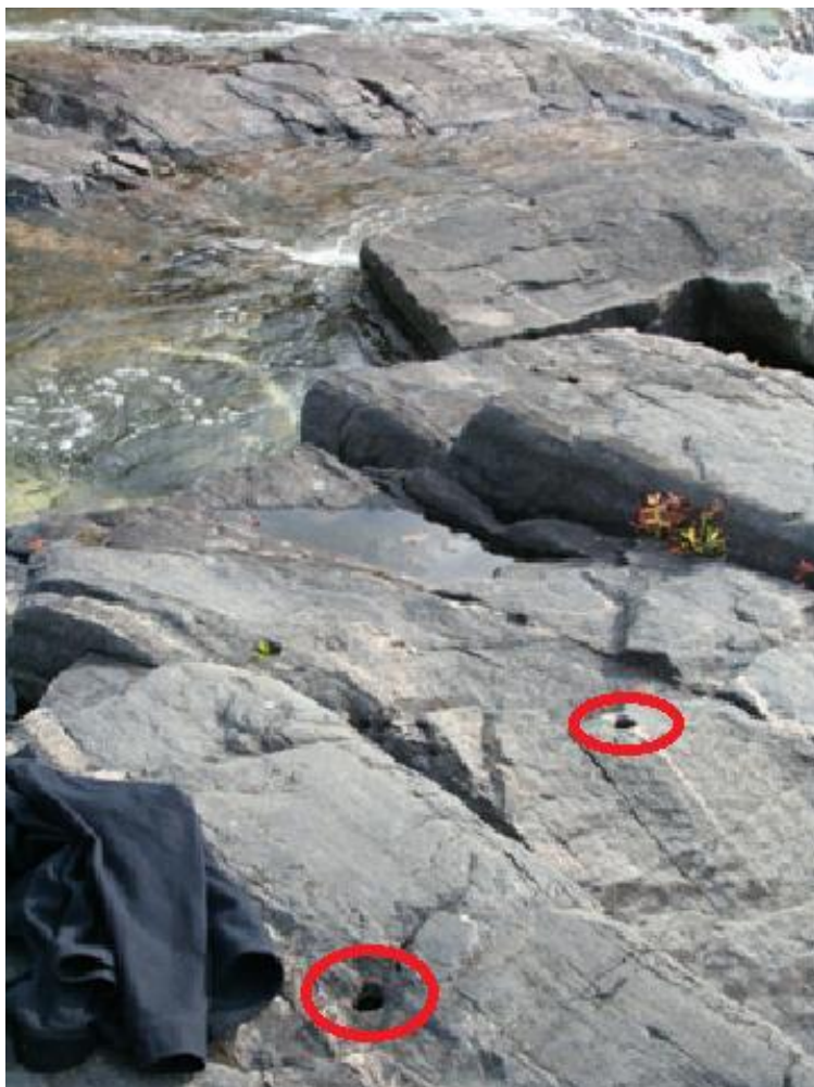
Photograph 5: Drill holes (indicated by red circles) for blasting charges in rock at the base of North Falls, 2012.
