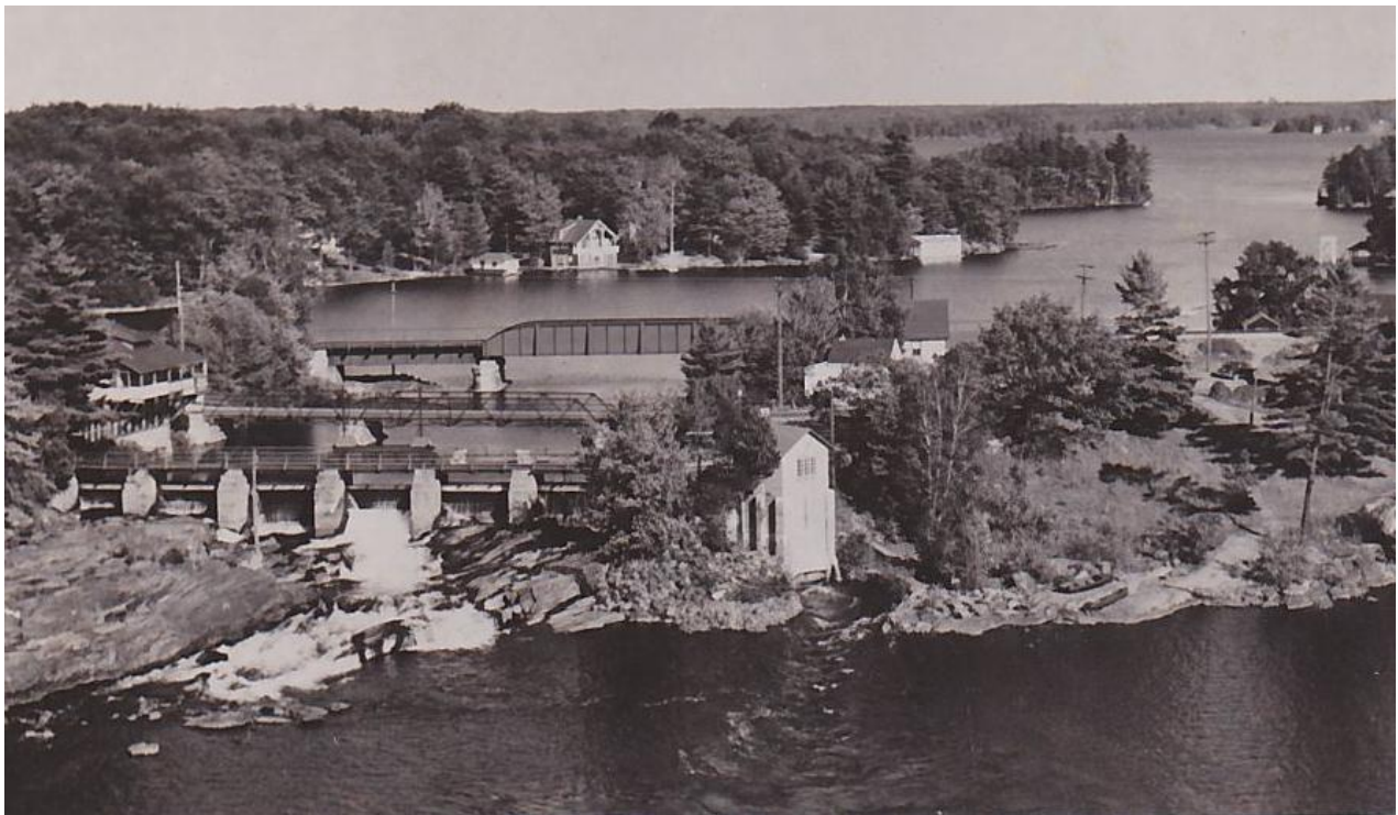
Photograph 1: Bala #2 Generating Station at the North Bala Falls, pre 1956.
