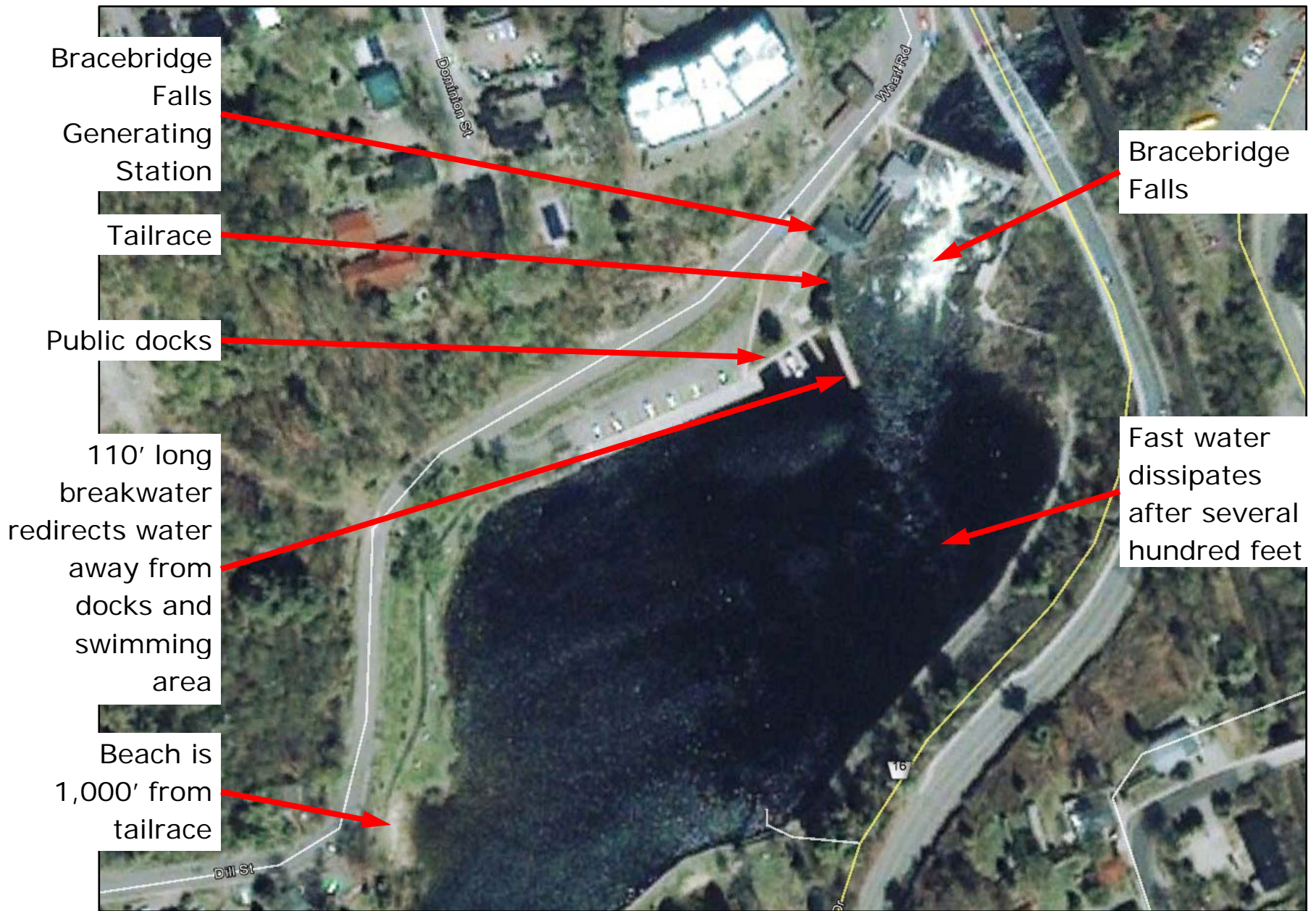
Breakwater protects boats and swimmers from the fast water from Bracebridge Generating Station
