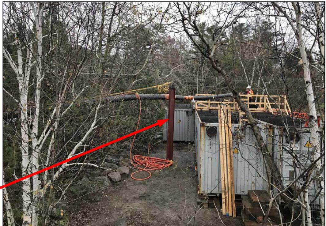
Suspended pipe cable is supported by steel post
