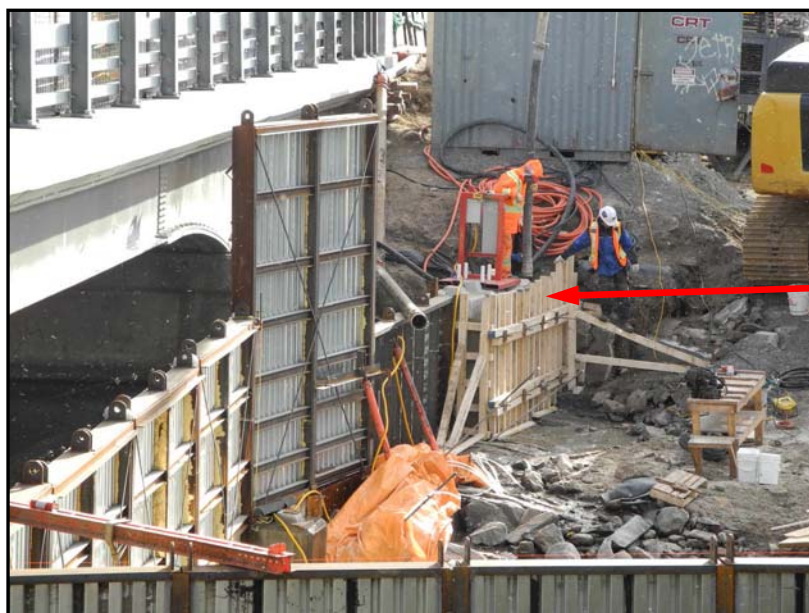
New poured concrete wall in Bala north channel, photograph taken 20171122
