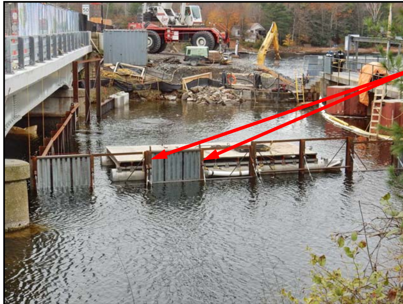
There are two non-removable steel channels for each removable panel, photograph taken 20171104
