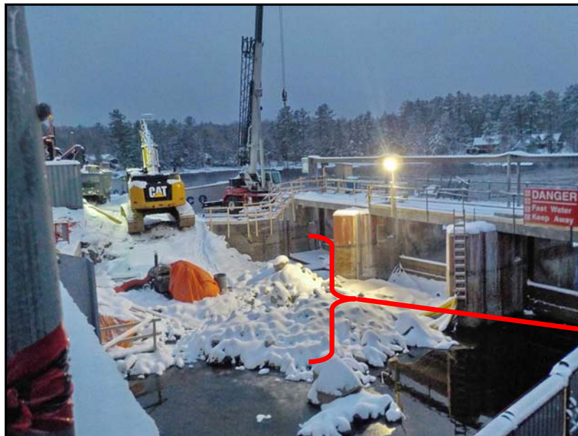
Rock debris in Bala north channel, photograph taken 20171207
