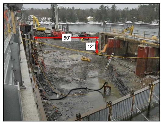
This temporary dam would need to be in place during the spring freshet, which is when the flow through the Bala north channel is the greatest and most unpredictable.
