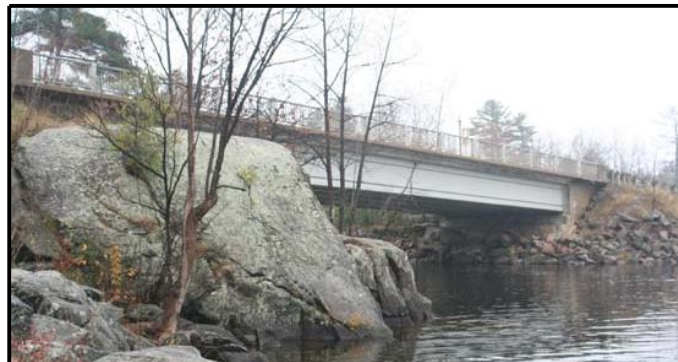
Figure 39 South Channel bridge showing bedrock of original shoreline on left and filled shore on right.
