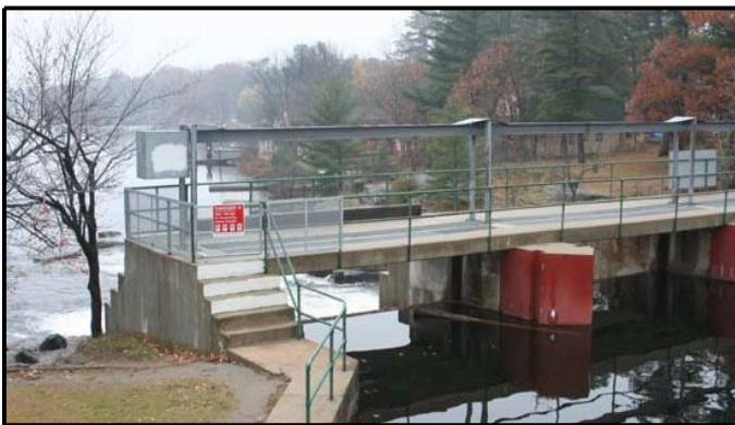
Figure 13 Looking downstream to the Muskoka River from the 1958 control dam.
