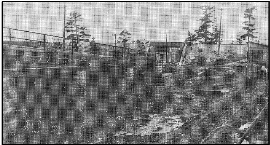
Figure 32 1913 bridge and dam under construction. The house visible through the railway underpass can be seen in Figure 20 Source: Petry, Bala
