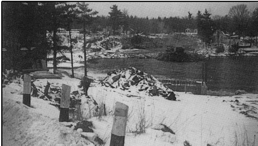
Figure 38 South Channel Bridge under construction showing land filling of bay. The old Presbyterian Church is in the trees on left. Source: Petry, Bala
