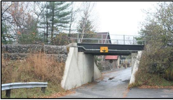
Figure 19 The single lane underpass with low headroom under the Canadian Pacific with the Presbyterian church in rear.
