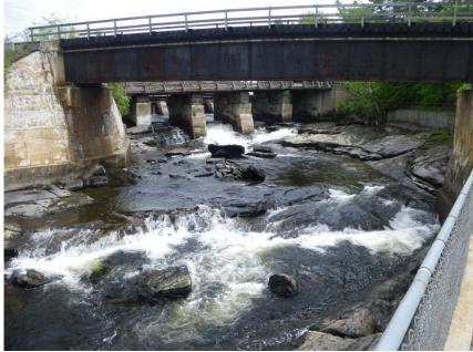
The above photos depict the minimum base flow (1 m³/s) to be passed over the South Bala Dam / Falls. Therefore, the flow passed over the falls will never be less than that shown above. It will, however, be greater than this during high flow times and specific high use periods as outlined in Table 2.
