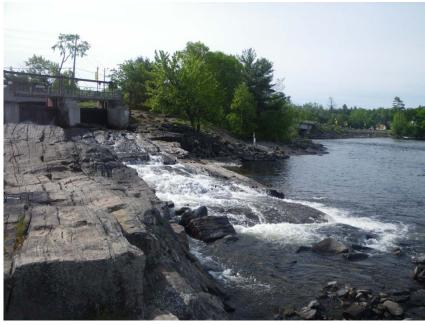
The above photos depict the minimum base flow to be passed over the North Bala Dam / Falls. Therefore, the flow passed over the falls will never be less than that shown above. It will, however, be greater than this during high flow times, walleye spawning, and specific high use periods as outlined in Table 2.
