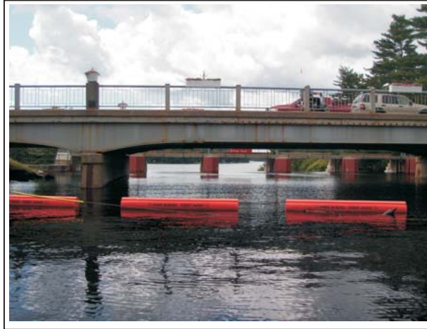
FROM UPSTREAM, DAM SHOWING OBSCURED DANGER SIGN
