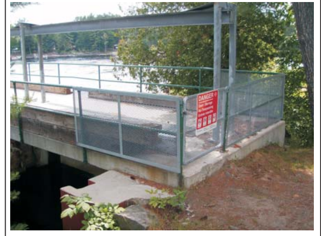
MESHED GUARDRAIL AND DANGER SIGN, NORTH END
