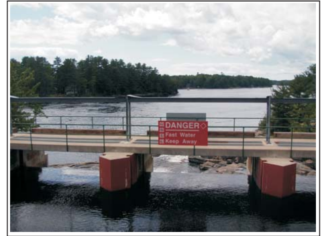
FROM HIGHWAY 169 ROAD BRIDGE SHOWING DANGER SIGN
