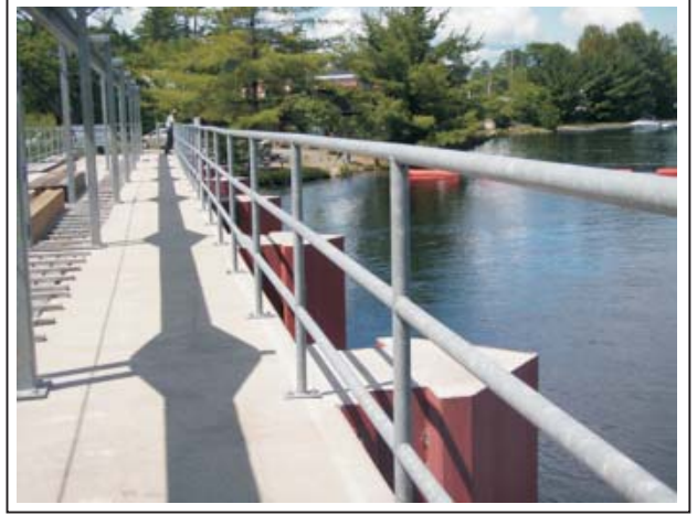
RAILING/BARRIER AROUND DAM DECK
